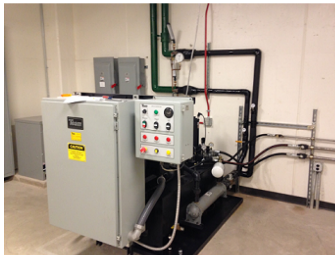
Figure 1.23. 3,000 PSIG hydraulic fluid is supplied to the VVA system in Test Cell #1 from a pump in the building's basement.
