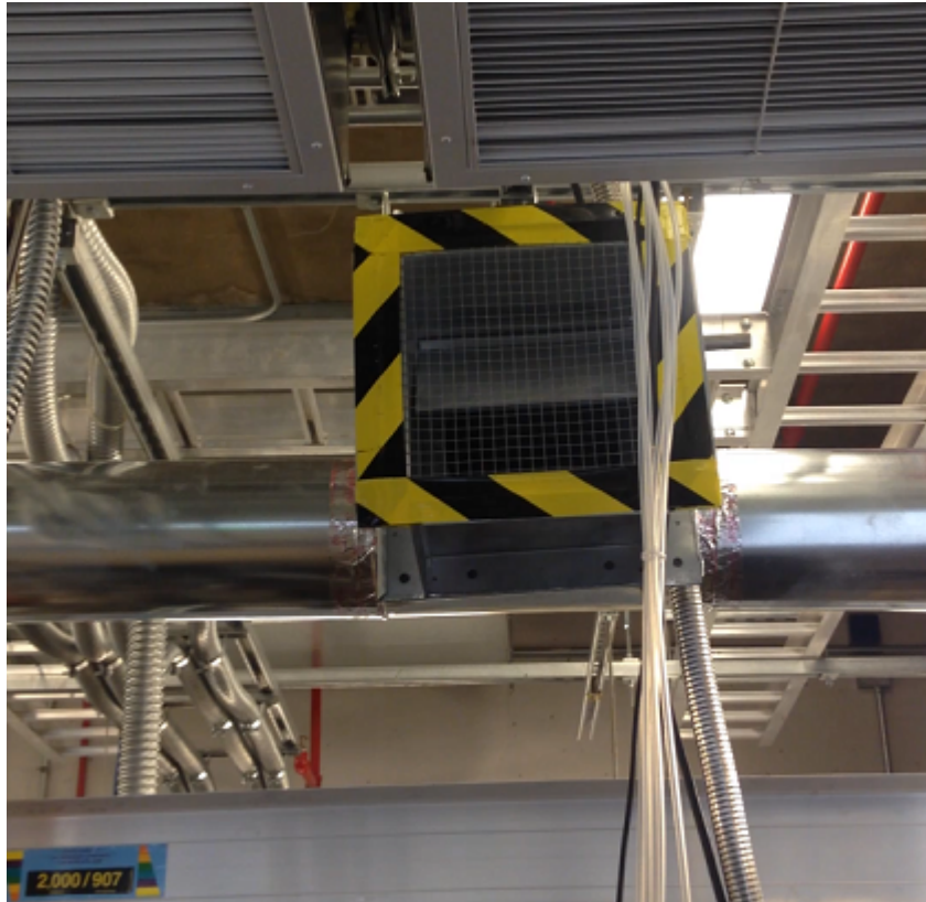
Figure 1.24. A weighted backdraft damper dumps excess air from the combustion air duct into Test Cell #1.
