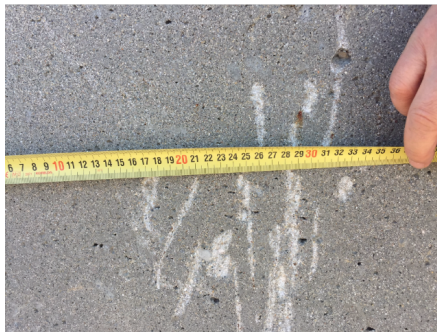
Fig. 4.75. Concrete Divider 4 rough surface (left) and broken surface (right)
