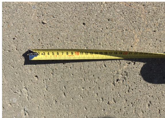
Fig. 4.73. The rough surface of Concrete Divider 4
