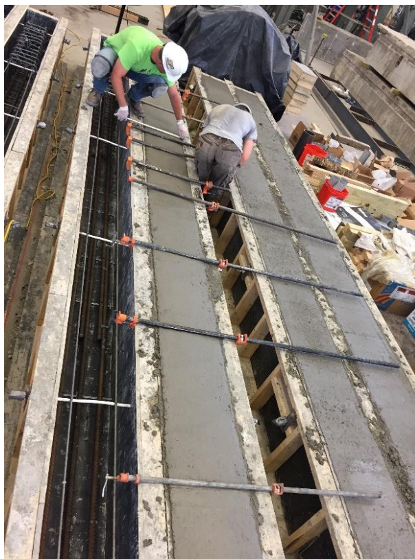
Figure 4.23: Series VI Form Bracing
