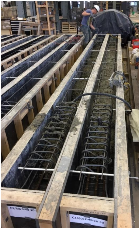
(a) Half-Beam Casting
