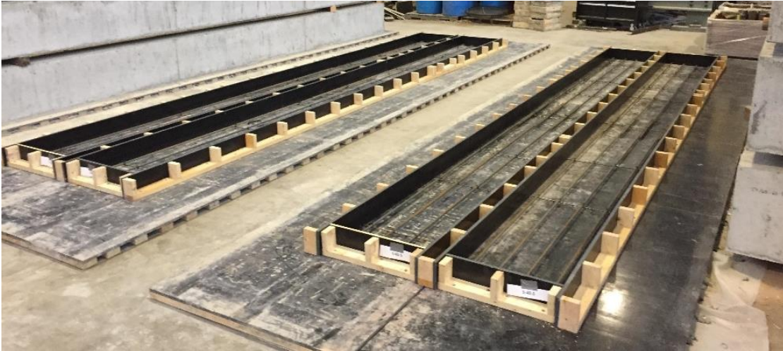
Figure 2.11: Series V Completed Formwork
