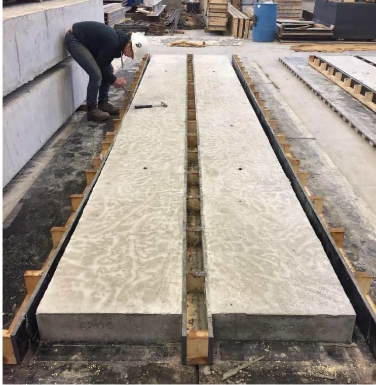
Figure 2.20: Series V Side Form Removal
