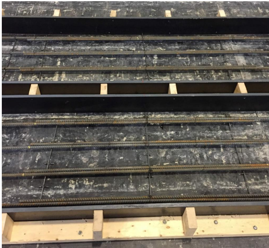
Figure 2.13: Slab Construction – Splice Region
