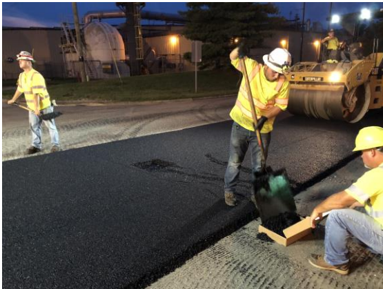
Figure 3: Sample collection at a Superpave 5 project site
