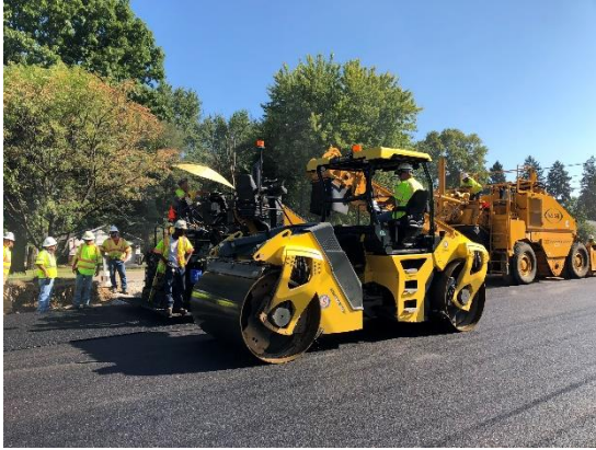
Figure 44: Compaction photographs for Project R 30280
