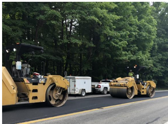
Figure 26: Compaction photographs for RS 39149
