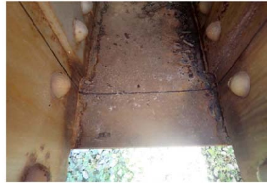
Photo 21: Bottom batten plate at Cross Section 3
