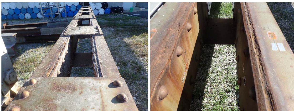
Figure 6.3 View of typical corrosion damage resulting in section loss and pack rust
