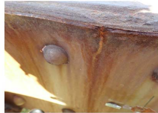
Photo 6: Crack in web plate near top (similar in a few locations)
