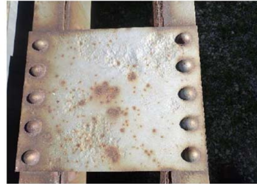
Photo 5: General condition of batten plates
