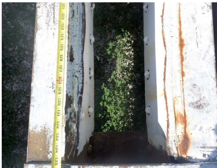
Figure 6.7 Truss chord near the critical section identified by three inspectors
