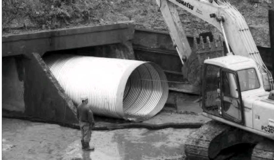
Fig. 1.3. Relining of a failed concrete box with corrugated steel pipe-arch [1].
