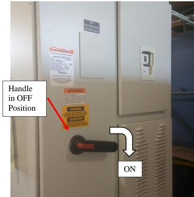
**Figure 4: Variable frequency drive**
