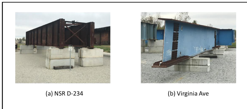
Figure 8: Steel bridge members at S-BRITE: (a) Norfolk Southern Railroad deck plate girder span; (b) Virginia Avenue bridge girder.
