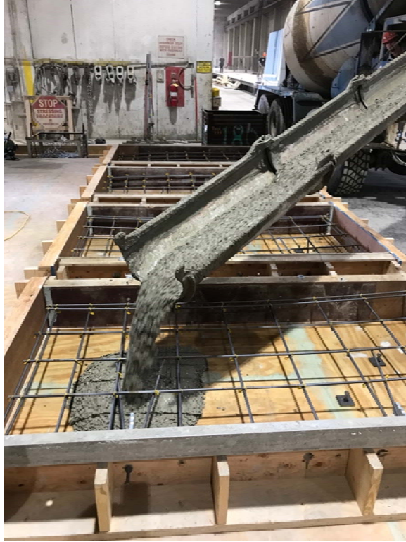
(a) Casting concrete
