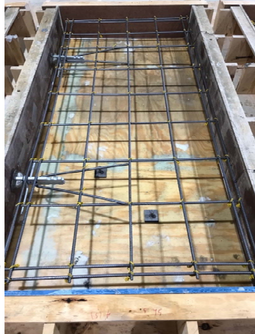
(b) Reinforcing bars and formwork
