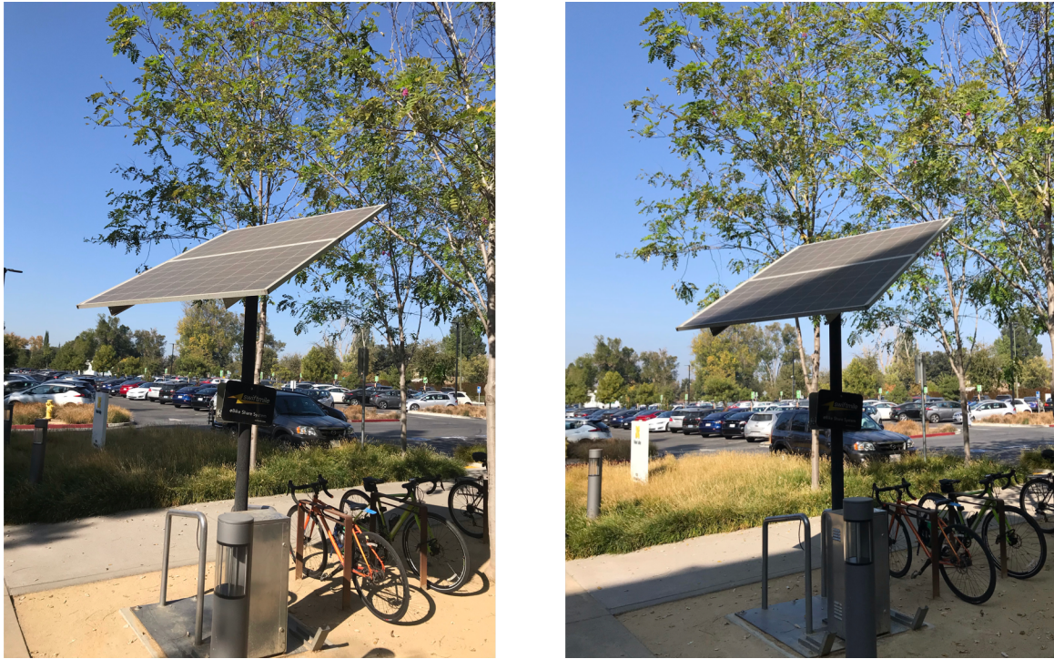
Figure 2.5. Shading Effect on PV modules: No shading (left) and shading (right)
