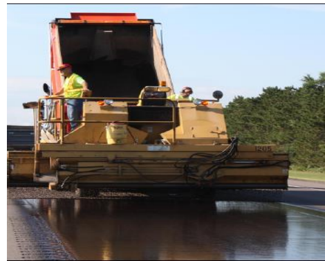
Figure 5.2. Chip Seal
