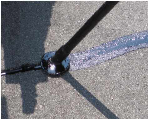
Figure 5.1. Crack Sealing
