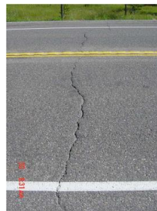
Fatigue cracking
