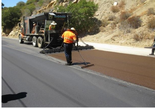
Figure 5.3. Micro-surfacing
