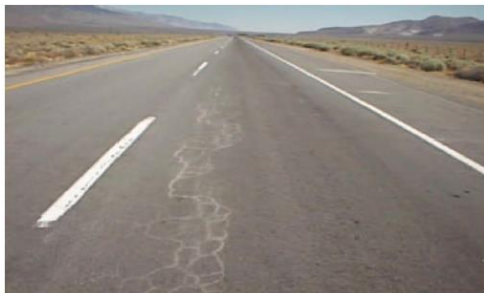
Fatigue cracking
