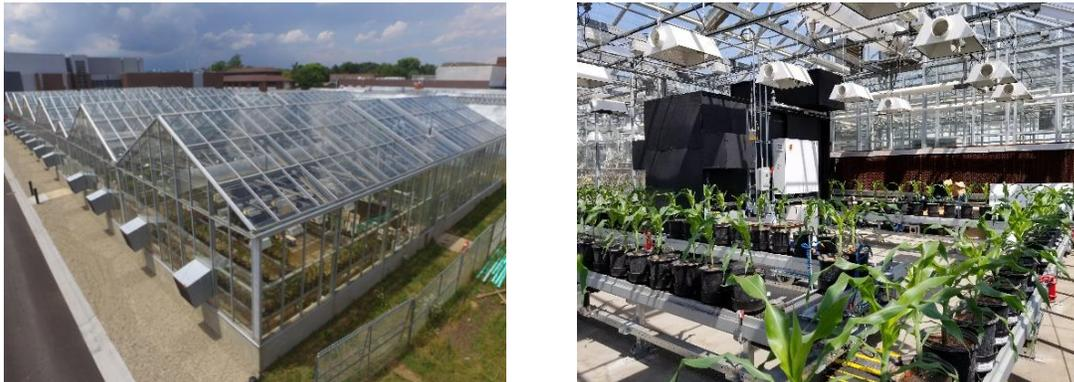
Fig. 3.1. Purdue Lily Greenhouse with an automated, high-throughput imaging system and a belt-conveyor-based plant transportation system.
