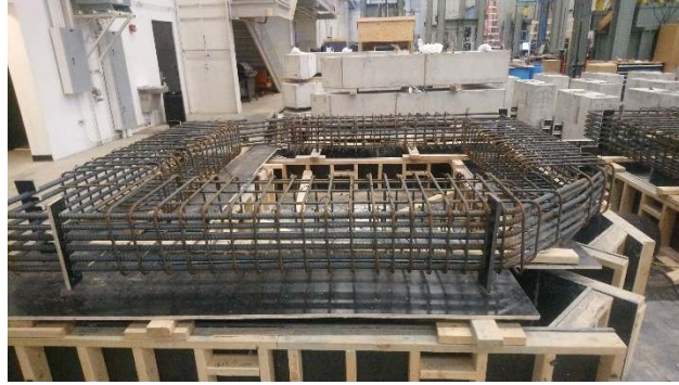
Figure 3-15 Construction of reinforcement cages
