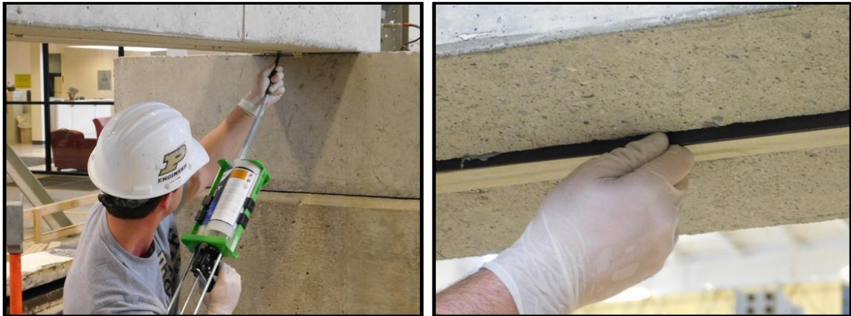
(a) Filling Groove with Epoxy
