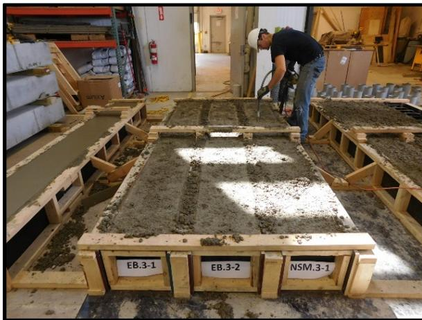
**(a) Vibrating Concrete into Place**
